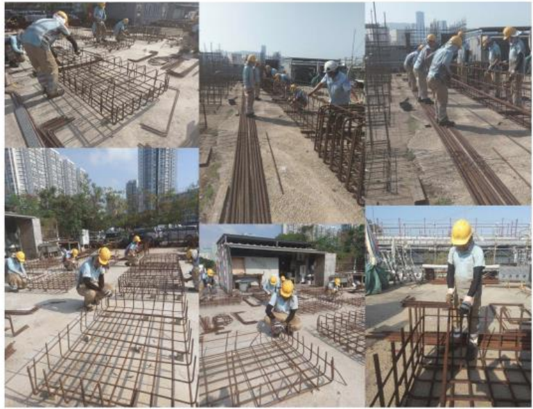
Figure 5. Bar bending and fixing tasks
