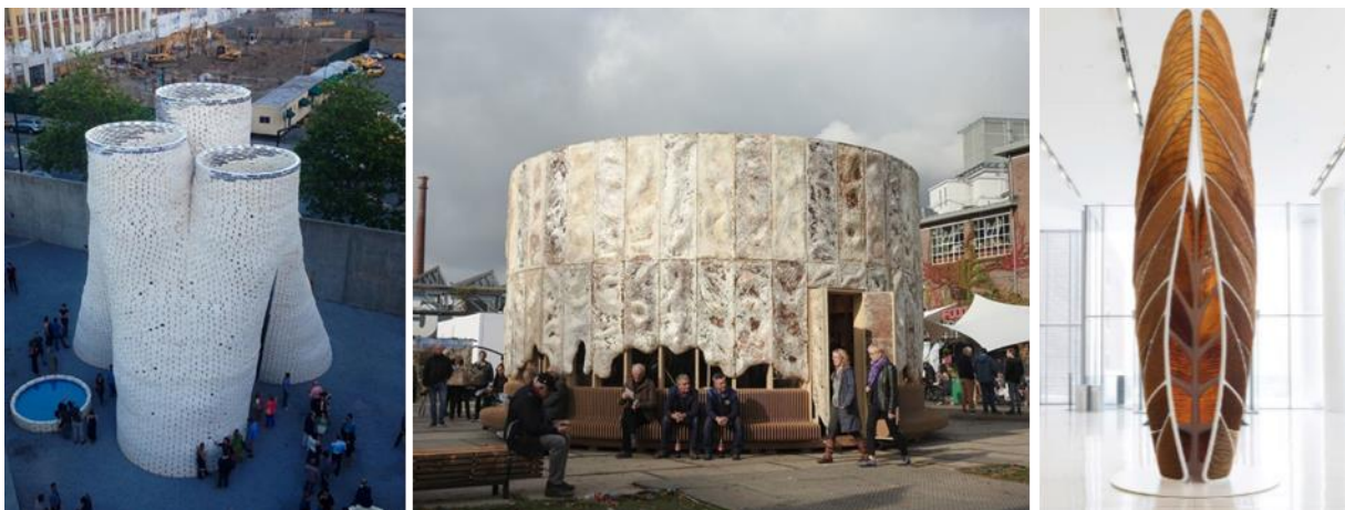
Figure 1. Hy-Fi Tower- Mycelium-bricks (left), Growing Pavilion Mycelium-panels (middle), Aguahoja Biopolymer Pavilion- Bacterial cellulose (right)
