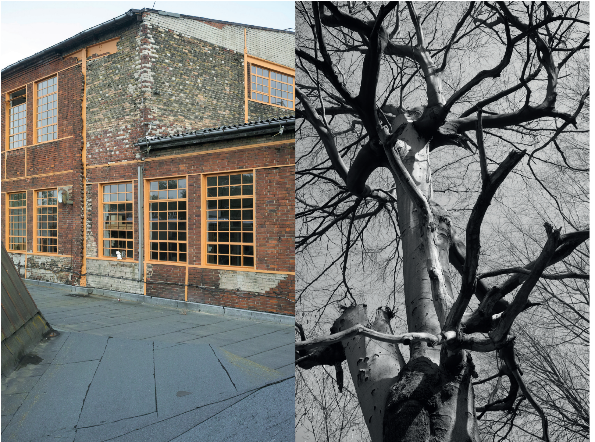
Photo: Silvan Linden, Energetic renovation and restructuring of Kunstfabrik am Flutgraben in Berlin; Old beech tree, Tiergarten.
