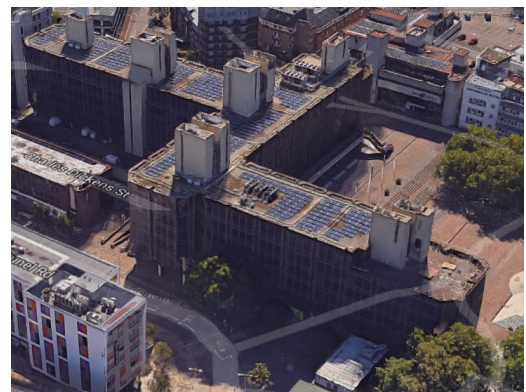
Figure 1: Portsmouth Civic Centre – (51)
