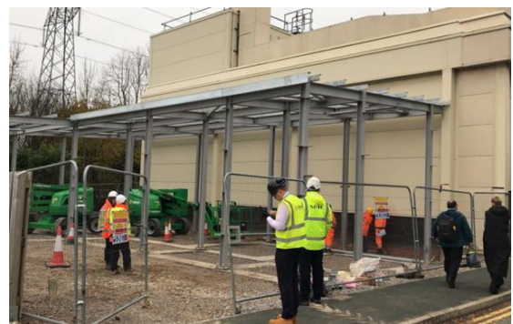
Figure 4. The safety zone selected around the steel erecting work to be monitored and controlled.
