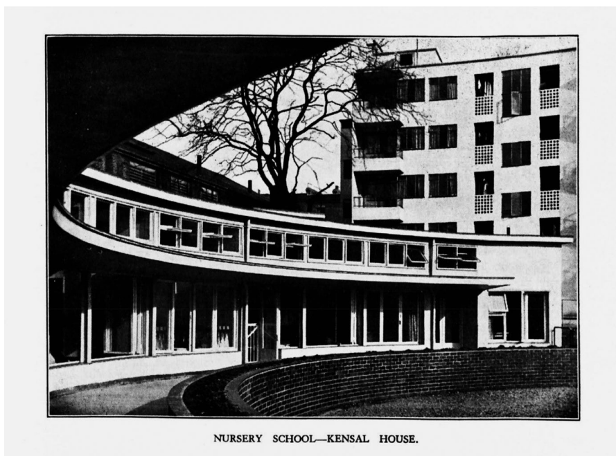
Figure 5. Kensal house and nursery school (Source: BL, Co-Partner's Magazine , Opening of Kensal House, April, 1937, p. 183).
