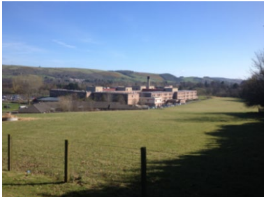
Figure 2. Haith Royal Infirmary - wrapped in carparks.
