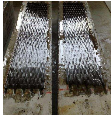
Figure 8 – Wet lay up CFRP application
