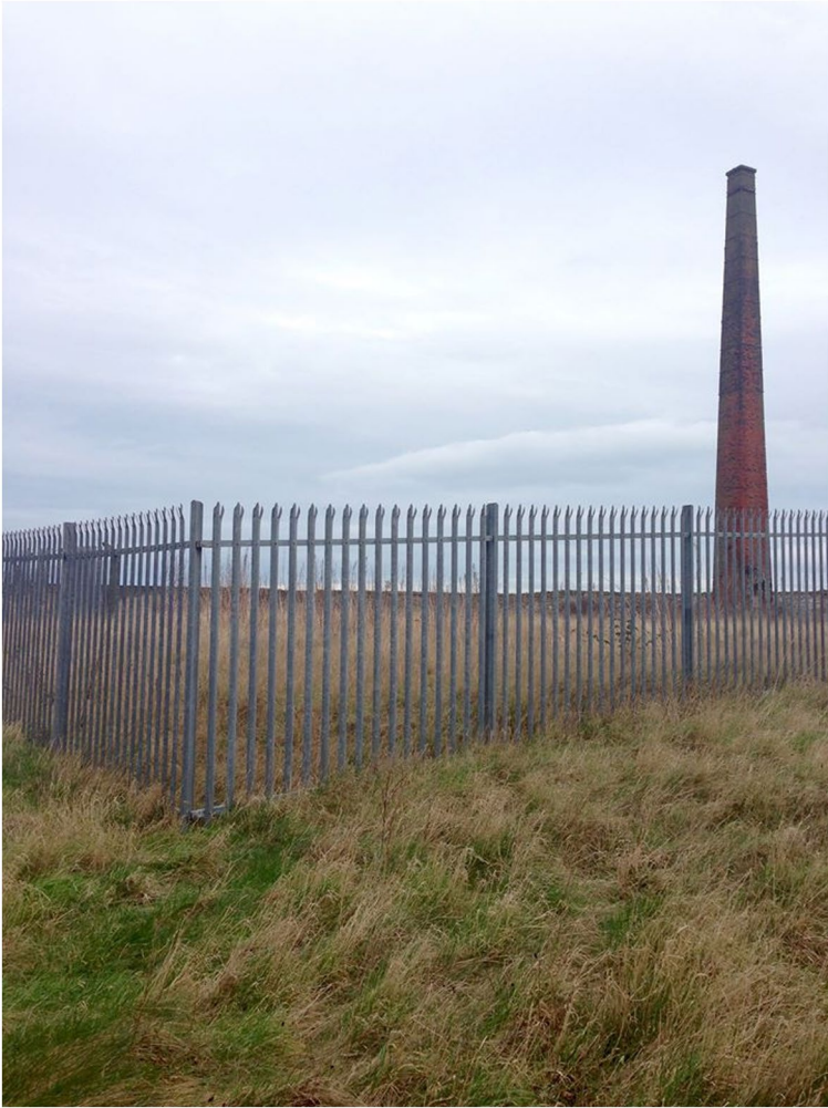
Figure 1: The chimney at Spittal Point. Photo: MG, 2016 [Colour figure can be viewed at wileyonlinelibrary.com ]
