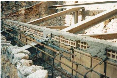
Figure 1. Example of a RC ring-beam.
