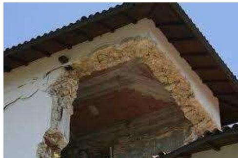
Figure 2. Example of an out-of-plane collapse due to poor connection between the RC ring beam and the underlying masonry.
