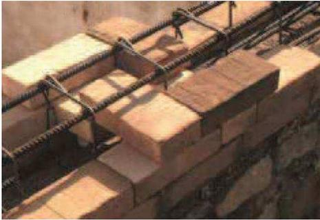
Figure 3. Example of a brickwork steel-reinforced ring-beam.
