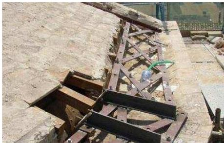
Figure 4. Example of a steel-profile ring-beam.
