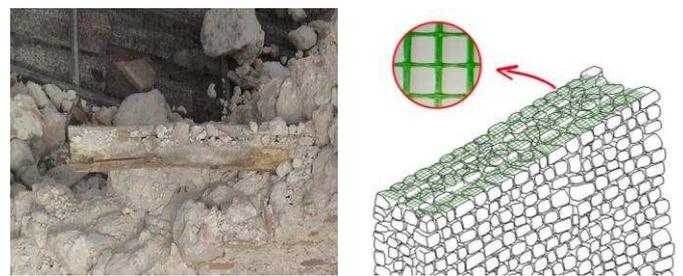
Figure 7. (a) Example of how a wooden beam is inserted inside masonry in an old building damaged by the L'Aquila earthquake in 2009; (b) Example of application of a GFRP grid.
