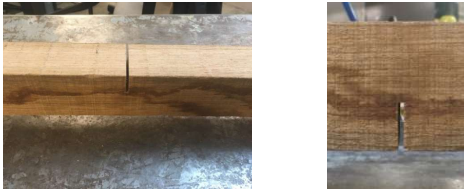
Figure 3. Damaged beam specimens (cut dimensions: 20 x 67 mm).
