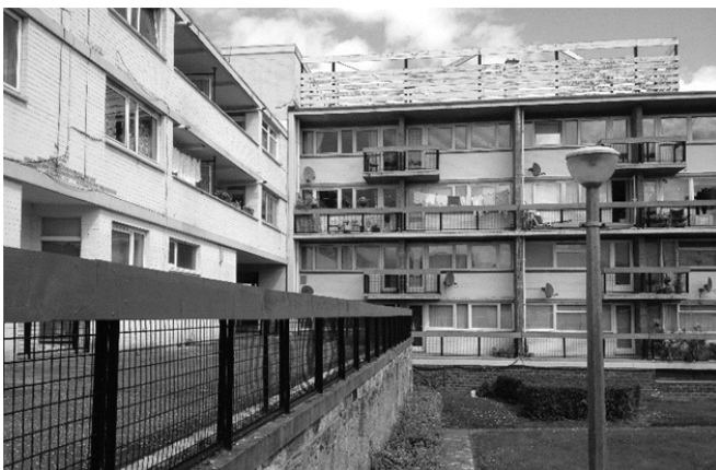
Fig. 5 Claremont Court. Block 3 and block 4 balconies facing the landscape courtyard. © Nadia Bertolino (2016).
