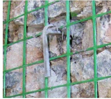
Figure 4 – Detail of the GFRP L-shaped bar
