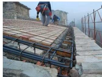
Figure 18 – Examples of reinforced concrete ring beams
