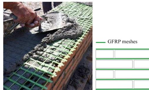
**Figure 21** – Clay brick FRCM ring beam
