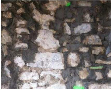
Figure 3 – Mortar joints repointed with new mortar
