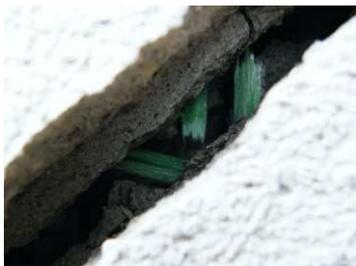
**Figure 10 – Detail of the GFRP mesh after cracking**
