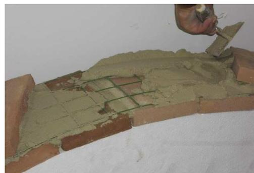
**Figure 15 – Detail of reinforced arch**
