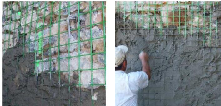
Figure 5 – Application of the mortar
