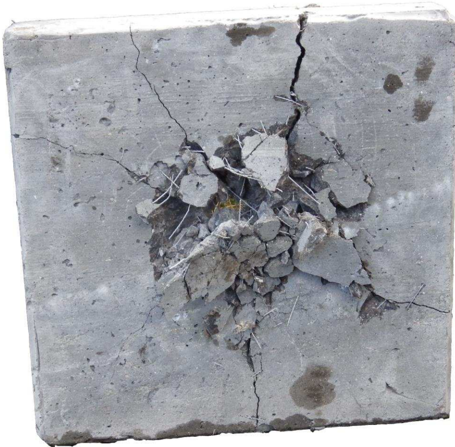
Figure 10 – Rear face of the Type 2 macro synthetic slab receiving multiple shots
