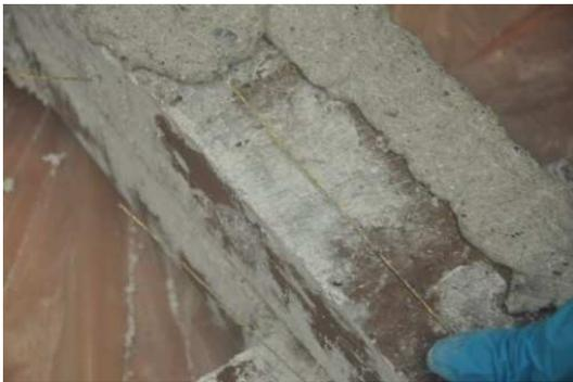
Fig. 16: Application of the steel cord in the horizontal mortar joint.
