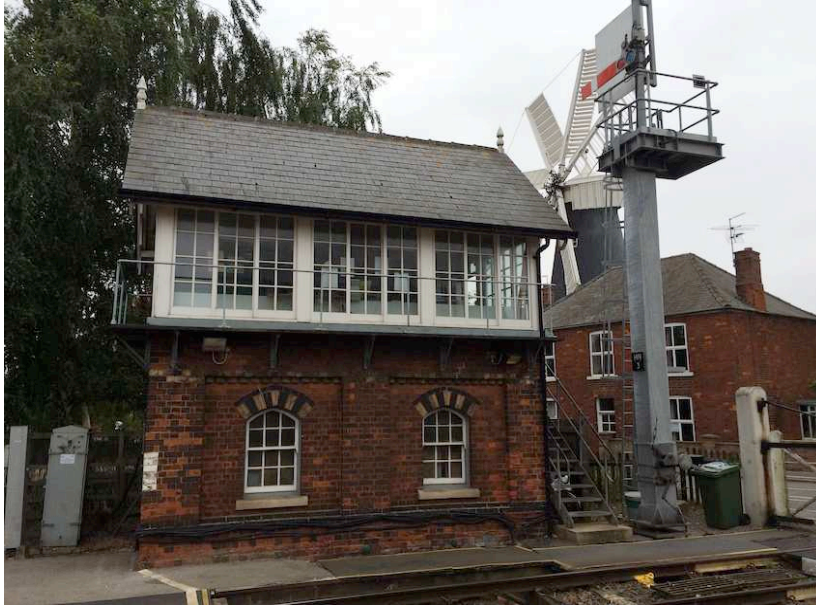
Figure 1: Heckington Signal Box (1876). This grade II signal box, with adjacent grade I windmill, almost represents an idealised English village environment. In this idealised world, the modern signal post is intrusive.
