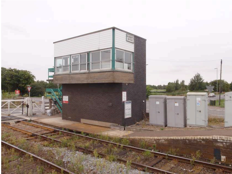
Figure 3: Hubberts Bridge Signal Box (1961). Possibly representing nearly the nadir of signal box design, this signal box is actually the next signal box along the line from Heckington. As an example of the era, arguably it is as worthy of preservation as it's prettier neighbour.
