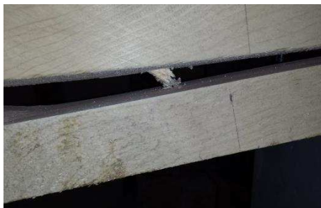
Figure 8. Pull out of the BFRP spike.
