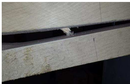
9 10 Figure 8. Pull out of the BFRP spike.
