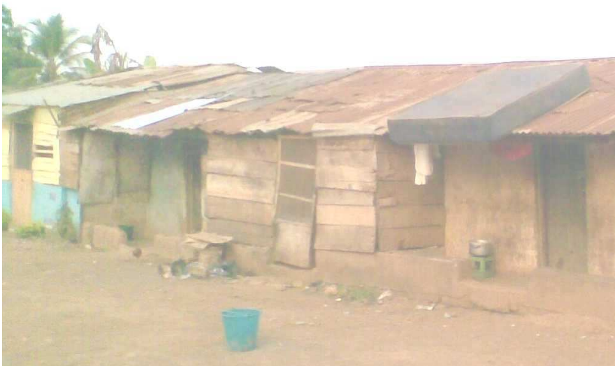
Figure 4: Houses with Reclaimed Timber Boards as Walls
