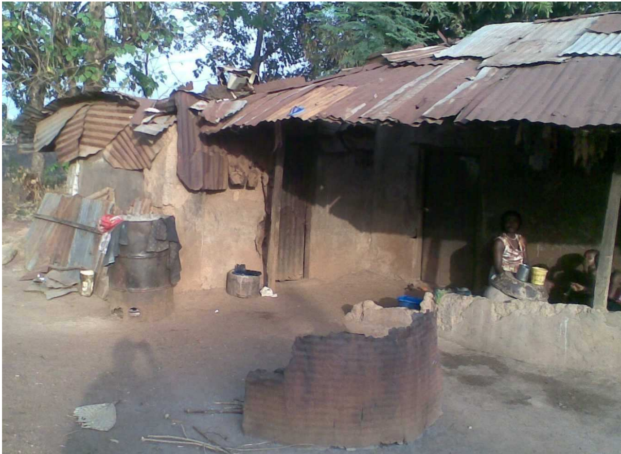
Figure 3: House with Rendered Clay Block Walls
