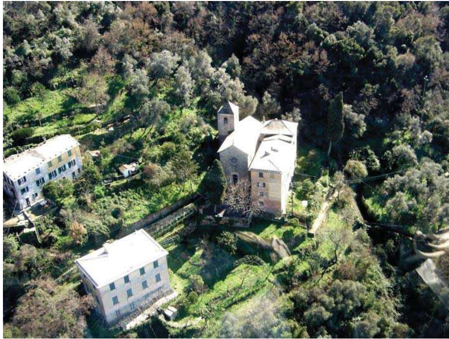
Fig. 2. Medieval church of Saint Nicolò di Capodimonte (Camogli, Genoa - Italy; author Arch. Paola Cavaciocchi)
