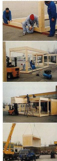
In systemised building, the quality and dimensions of individual components are defined by the relevant standards with a view to achieve optimised working procedures, but, in a way, limiting the degree of design freedom.
