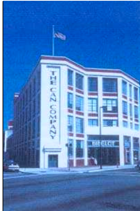
Figure 10: Signature Building, Norton Tin Can and Plate Company, Baltimore, Maryland
