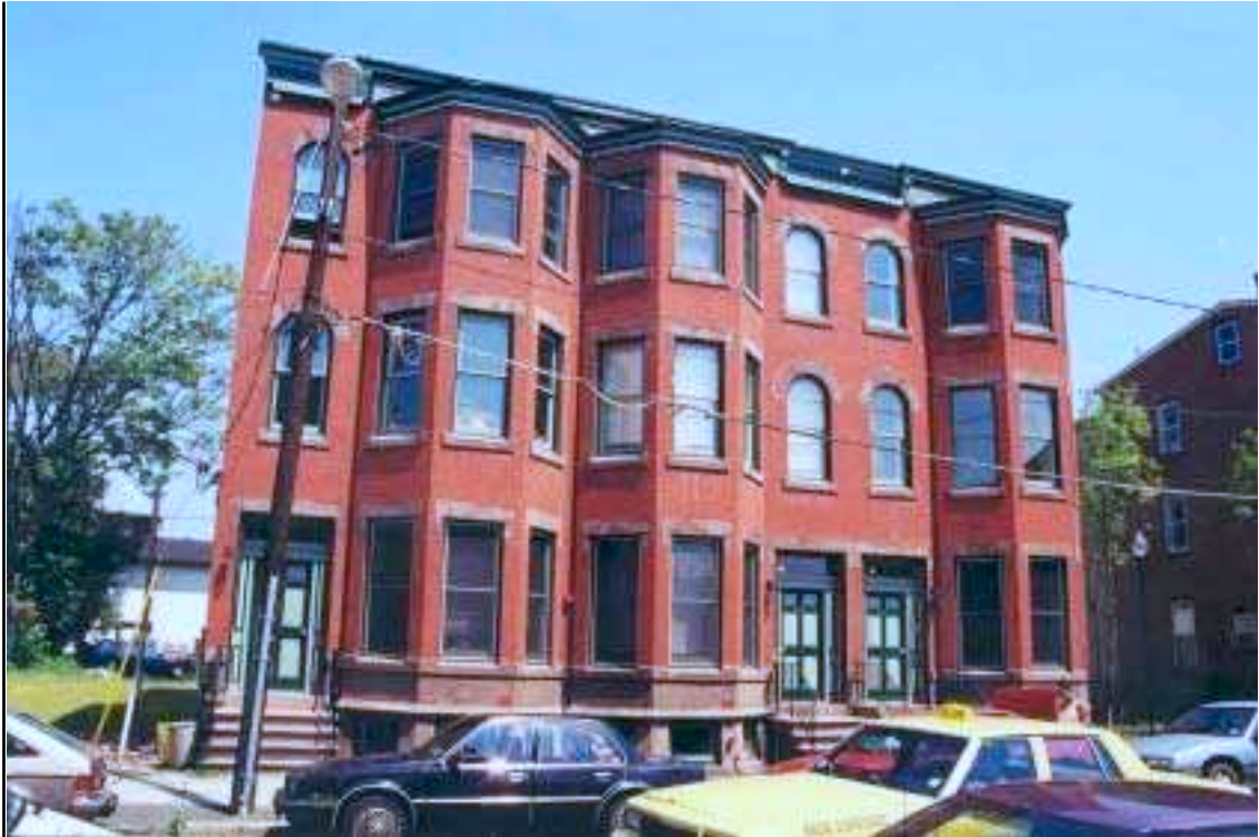
Figure 6: Rehabilitation of No. 210 Academy Street, Trenton, New Jersey (Academy Hanover Historic District): a timber frame and brick residence, constructed in circa 1900. The project involved the conversion of a single residence to two low-income residential units with the assistance of the both 20% federal historic rehabilitation tax credit and the low-income housing tax credit.
