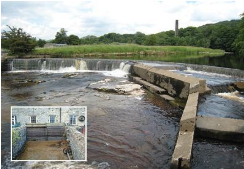
Figure 2: The Settle scheme. Source Settle Hydro.
