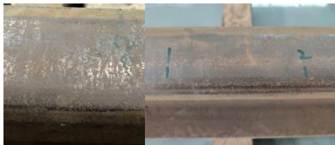
Fig. 16 Closed cracks (After rolling).
